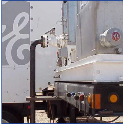
Liquid Fuel Supply (2" pipe)
