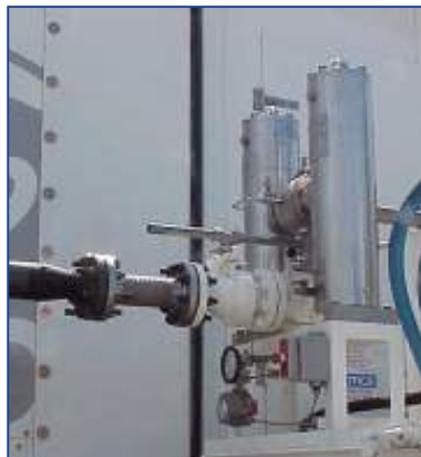
Liquid Fuel Supply (2" pipe)
